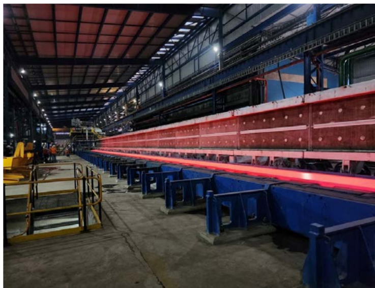
The new hot-strip mill complex makes use of many modern technologies, from melting through finishing
